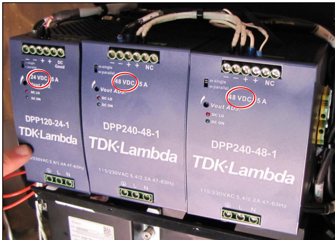
Figure 1-1: Power Supplies Unit
