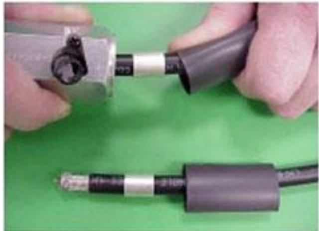
**STEP 4:** Debur the center conductor using the DBT-01 deburring tool.
