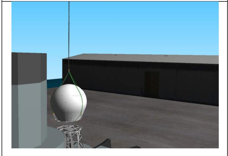
**STEP 4:** Insert M16 bolts, washers and spring washers downwards through the 10 lifting points on the ADE Base Ring, and tighten securely using appropriate nuts.
