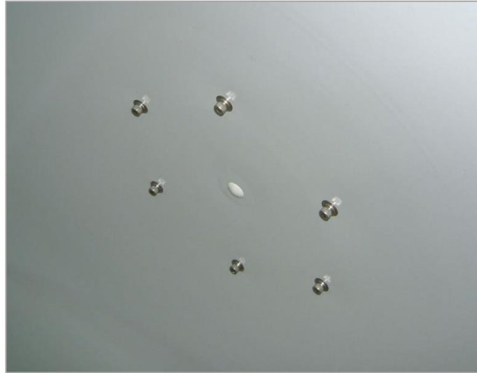
Figure 71. Antenna Assembly Installation
