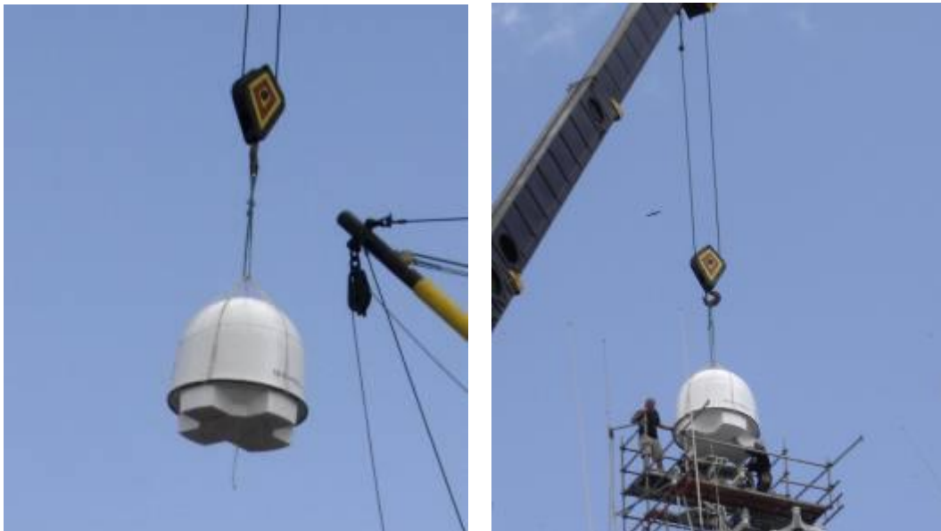
Figure 65. Lifting the ADE
