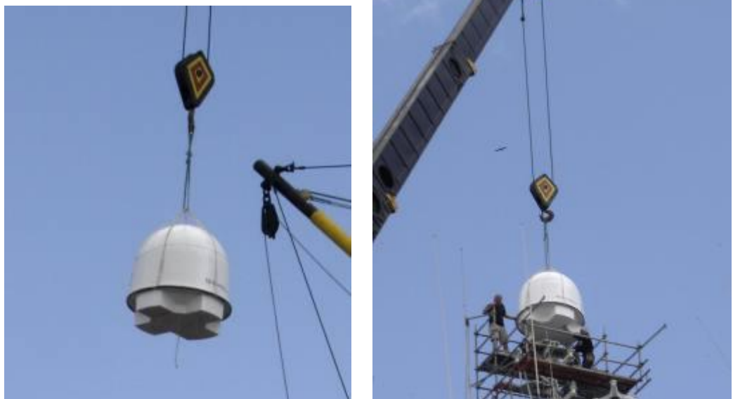
Figure 7-7. Lifting the ADE
