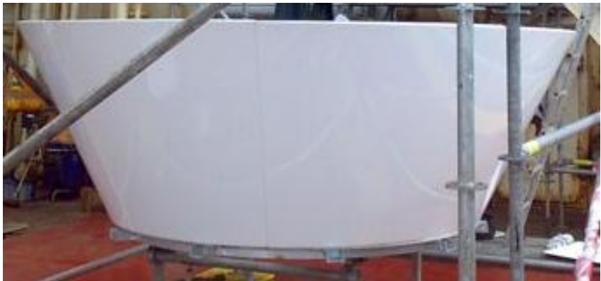
Figure 9-18: Lower Radome Section Secured to Radome Base
