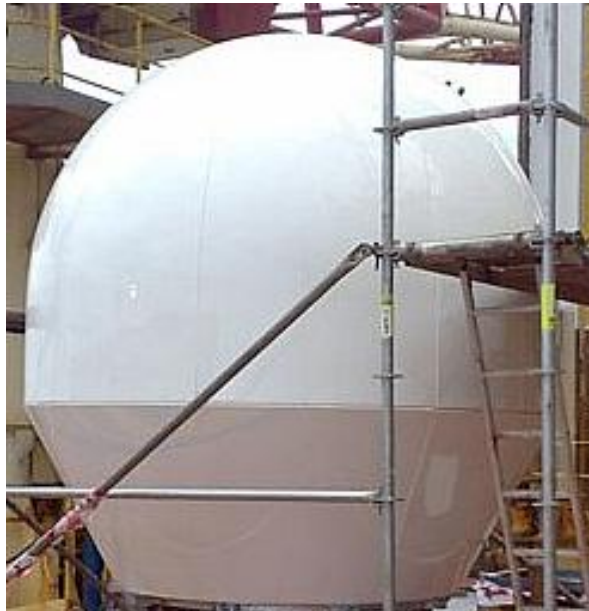
Figure 9-37: Lowering the Radome Upper Section onto the Lower Section
