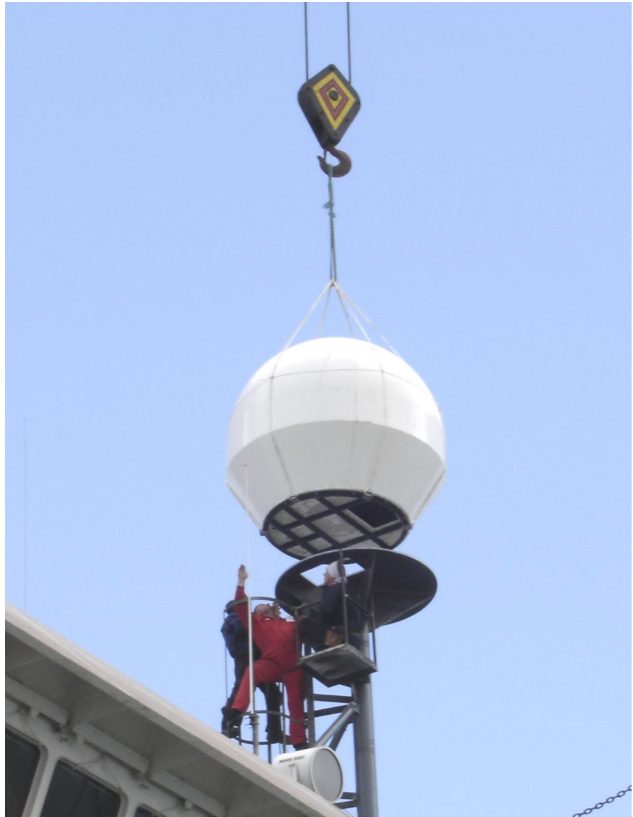
Figure 9-44: Lifting the ADE onto the Support
