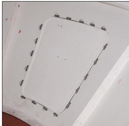
Figure 9-19: Hatch viewed from the inside
