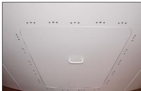
Figure 9-20: Hatch viewed from the outside
