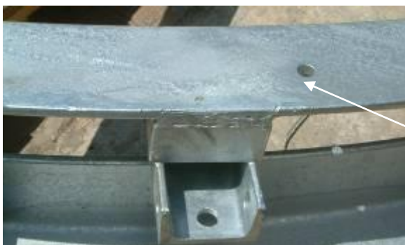
Figure 9-17: Base Ring Mounting Holes
