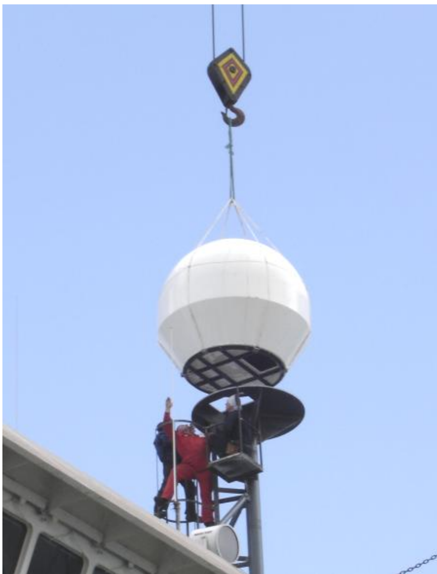
Figure 9-44: Lifting the ADE onto the Support
