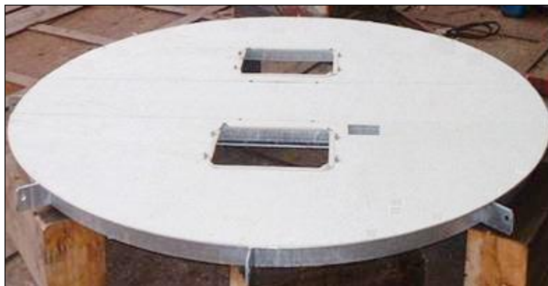
Figure 2-8: Radome Base Floor Secured to Base Ring
