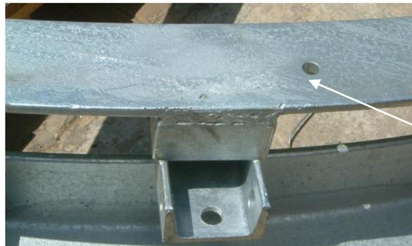
**Base Ring Mounting Hole for the Radome Base**
