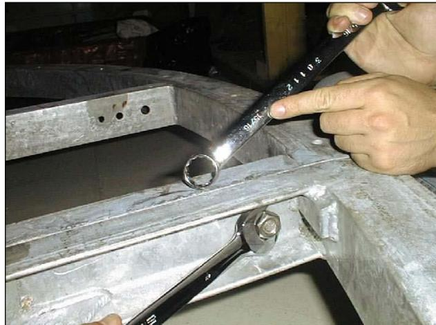
**Figure 9-3: Assembling the Base Ring**
