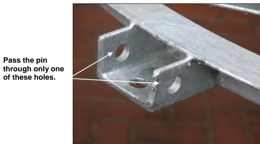
Figure 9-32: Lifting Point
