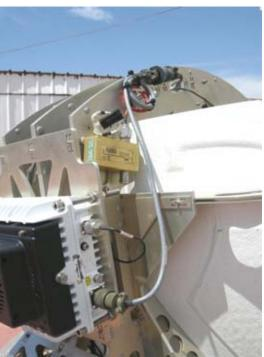
**Step 6**Bind the cables to the DISH ASSEMBLY with tie-wraps.
