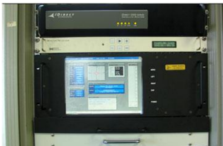
Figure 10-4: Typical BDE rack installation
