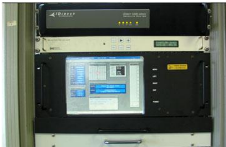
Figure 10-4: Typical BDE rack installation
