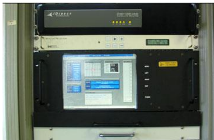
Figure 10-4: Typical BDE rack installation
